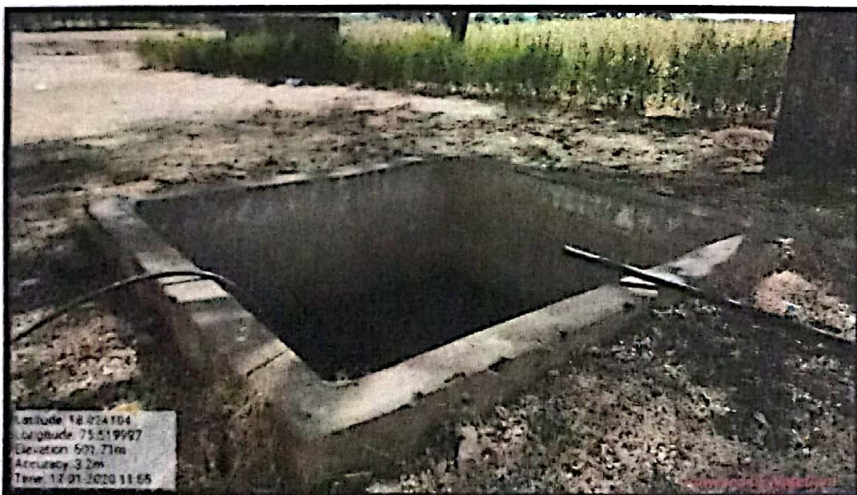
TANK FOR WATER STORAGE
